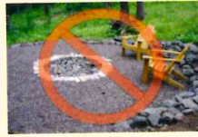
This fire pit does not have containment above grade level.
